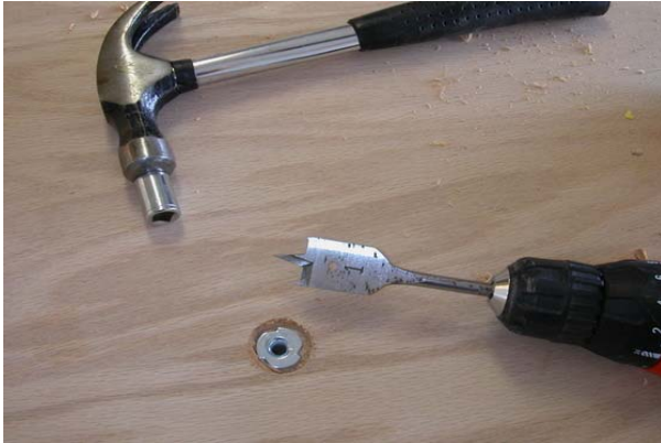
Drilling a pilot hole on the rail.
